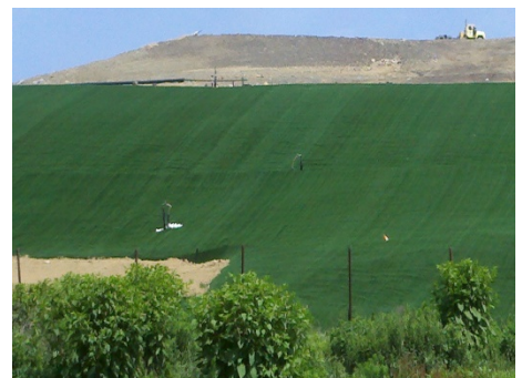
A side slope installation of Closure Turf integrating existing vertical wells
